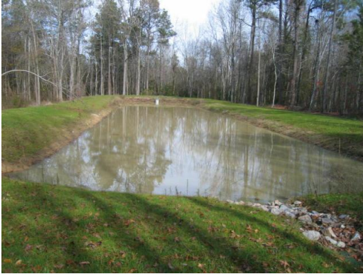
Wet Detention Pond
